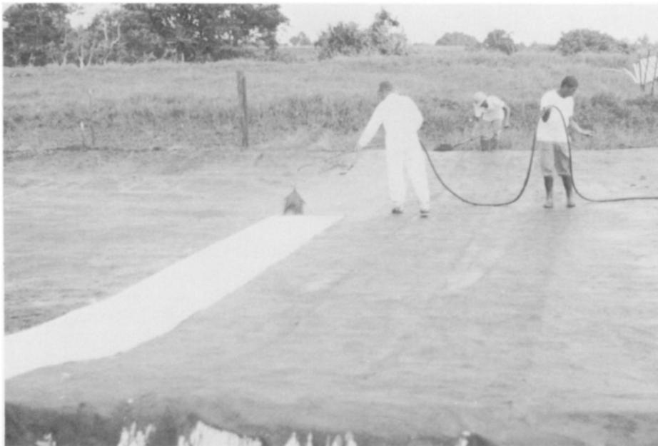
Fig. 4. Laying the fiberglass mat and spraying with asphalt emulsion.
