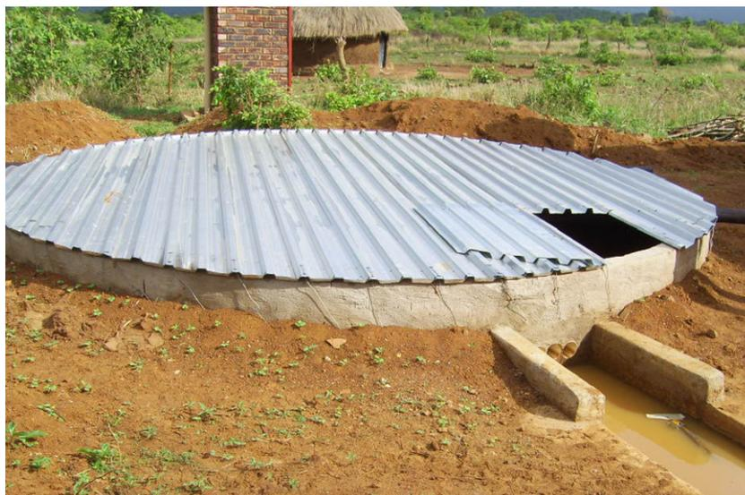
Fig. 1. 30 m<sup>3</sup> RWH underground tank constructed by under the DWAF demonstration phase (Picture by Papenfus).
