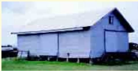
Pesticide storage shed
