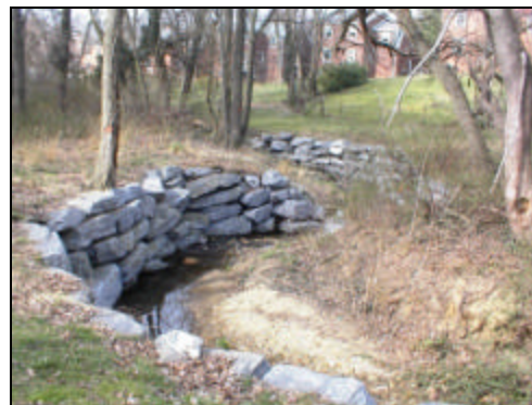
Imbricated Rip-Rap - A highly structural stabilization technique used where erosion potential is high and vegetative techniques are not likely to be effective.
