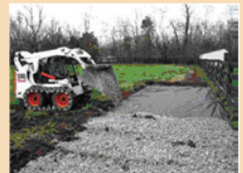
Figure 5. Base layer of crushed stone.
