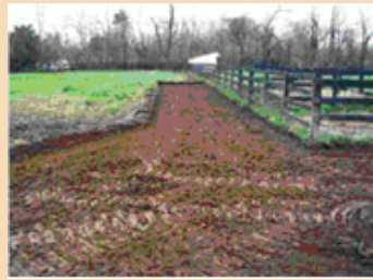
Figure 2. Excavation through the topsoil to stable soil beneath.
