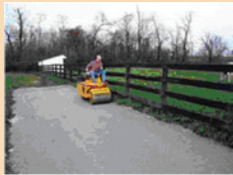
Figure 9. Compaction with drum roller.
