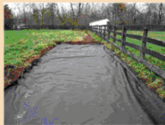
Figure 3. Geotextile fabric in place after excavation.
