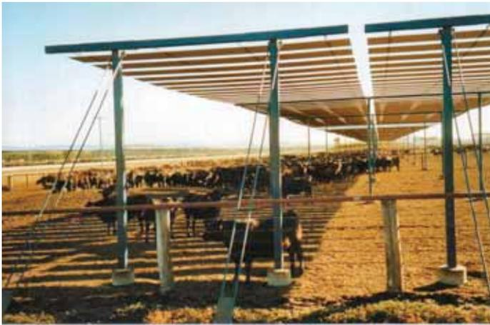
Figure 2: Feedlot iron sheet shade structure
