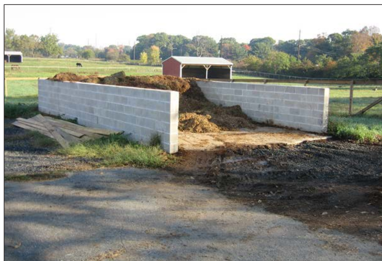
Figure 23. Dry stack manure storage area. Photo courtesy of the Livestock and Poultry Environmental Learning Center.
