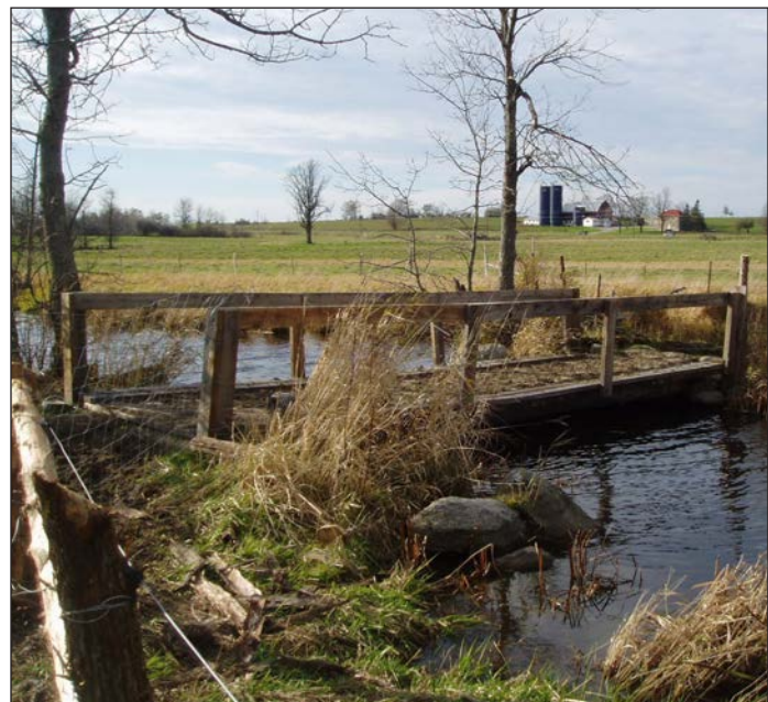
Figure 17. Above-water cattle crossing structure. Note the unaffected adjacent stream banks. Photo by Garnet Baker.
