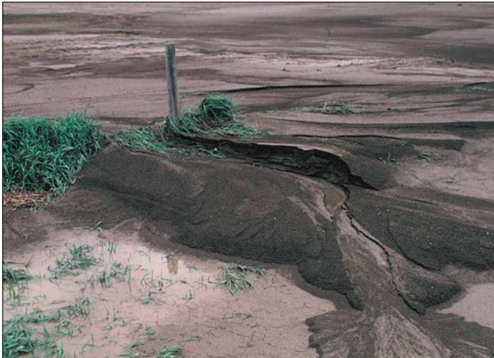
Figure 6. Typical erosion due to unprotected soil. Photo by Lynn Betts, USDA–NRCS.
