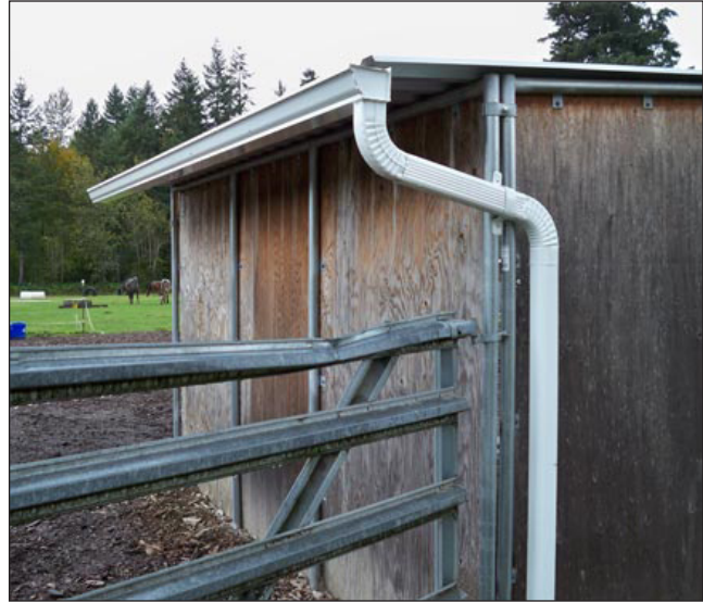
Figure 13. A roof runoff structure like the one pictured helps collect, control, and transport precipitation from roofs. Photo courtesy of the King Conservation District.
