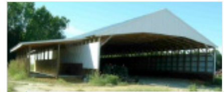
Manure storage shed. Photo courtesy of TJ Farms.
